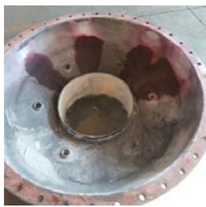
Vessel head weld repair
