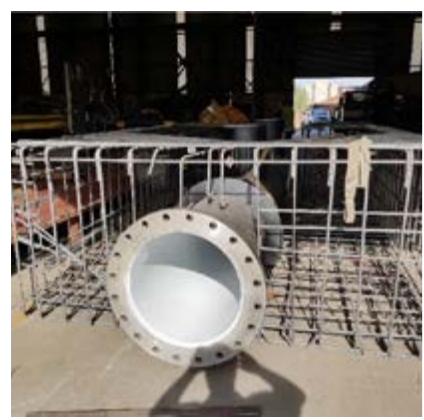
Penstock Inlet for fine ash dam
