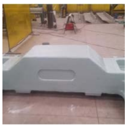
Plate mill pressure casting repair
