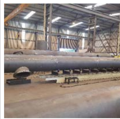
CO2 Gas line for steel coke ovens
