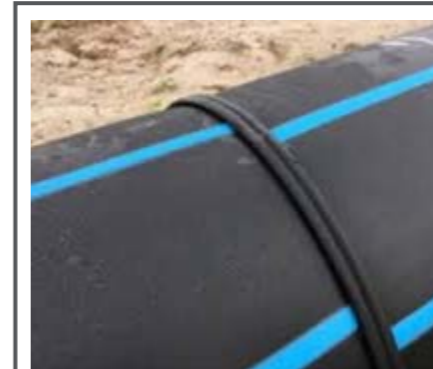
HDPE field weld
