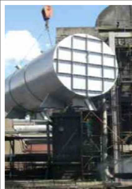
Installation of 600mm Dia CO2 pipe line to coke ovens
