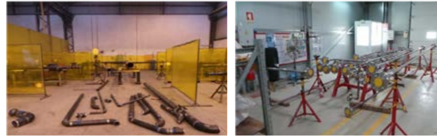
Welding bays for Carbon and Stainless steel (SEGREGATED)
